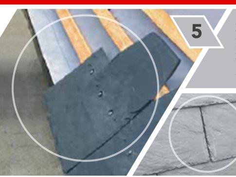
Once all the underlay and battens have been fixed into place cut the eaves slates to a length of 300mm by using a hand saw or similar. If it is a straight up and over roof start at the verge allowing the correct overhang on the verge and the 50mm over the fascia/ eaves ventilation. Fix the eaves slates into the batten using the appropriate nails/screws.
